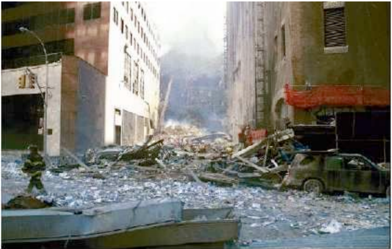
View from behind WTC 7 (northwest corner of WTC 7 is at left) from Barclay Street, looking towards WTC 6. Verizon building is at right. Note the size of the ejected column in the foreground compared to the fireman. Avery claims that building 7 was "barely even in the damage range."
